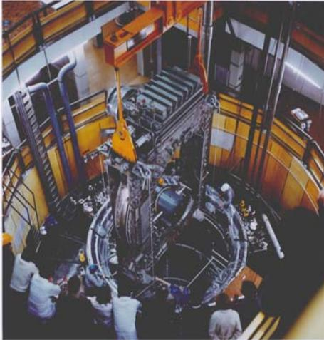
**Fig. 3.** Installation of the EURATOM LCT coil in TOSKA.
