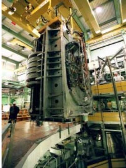
**Fig. 11.** Installation of the ITER TF Model Coil in TOSKA
