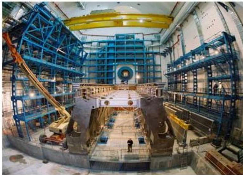
Fig. 3. The large ATLAS cavern in March 2004, ready to receive the ATLAS toroid. In the center, the tunnel of the LHC machine is also visible.
