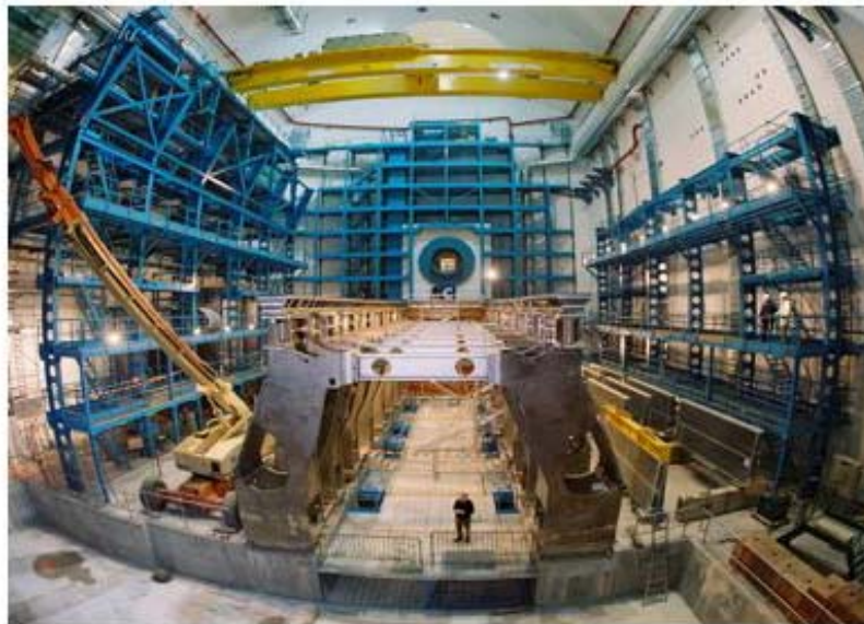
Fig. 3. The large ATLAS cavern in March 2004, ready to receive the ATLAS toroid. In the center, the tunnel of the LHC machine is also visible.
