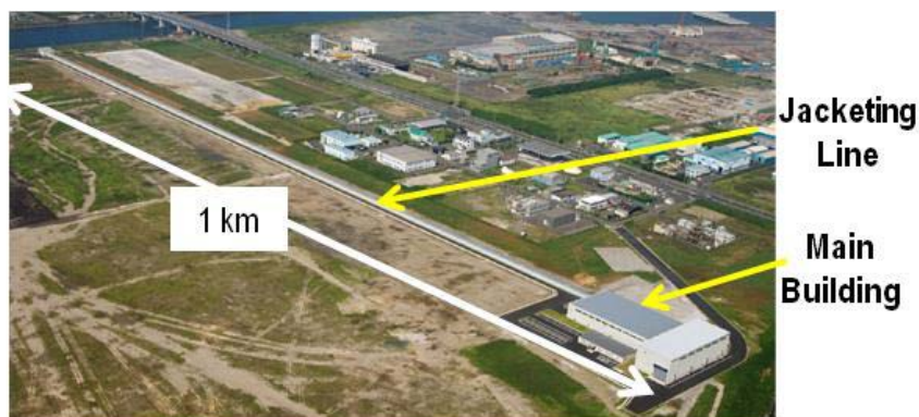
Fig.14. Aerial view of the 1km-long jacketing facility for the ITER conductor (Courtesy of Japan Atomic Energy Agency) [26].
