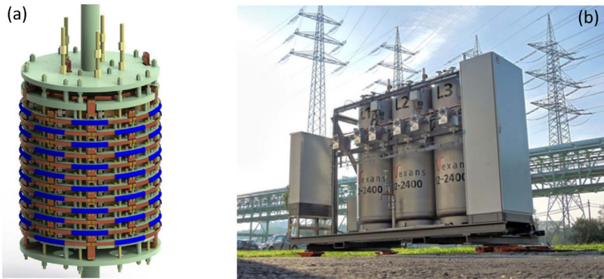
Fig. 22 (a) 3D CAD model of an actual R-SFCL designed for the ECCOflow project [167]. (b) The R-FCL installation of the AMPACITY project [168]
