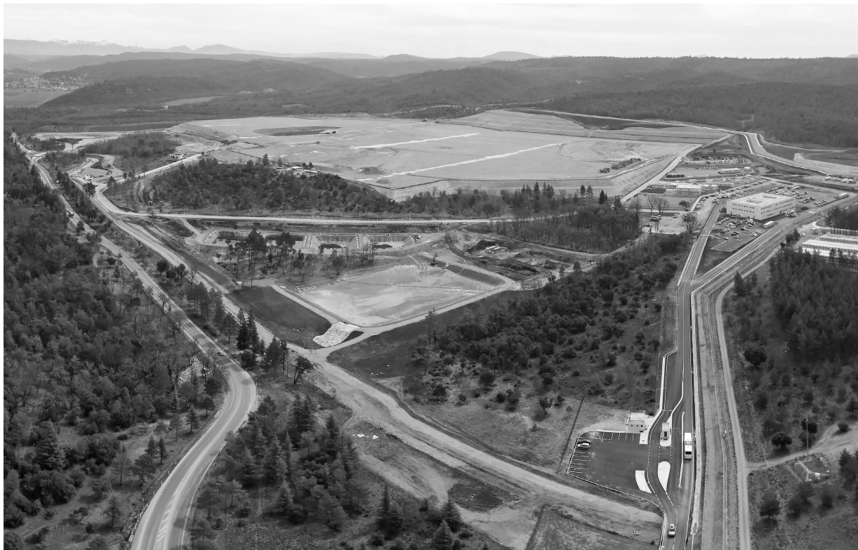
FIGURE 1. Status of the ITER construction site at Cadarache in April 2009.
