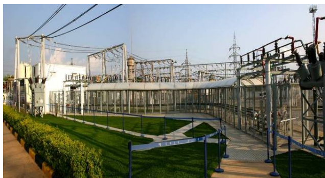
Fig. 15. The overview of the 35 kV/121 MVA cable installation site.
