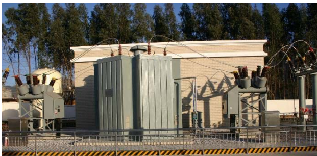
Fig. 18. The installation of 35 kV/90 MVA SISFCL.
