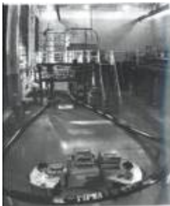
Fig. 2 (a). LTS power cable 50 m long developed at VNIKP.
