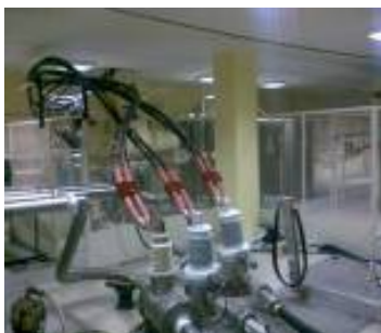
Fig. 13 (a). The 30 m cable: terminations of three phases at the test facility.
