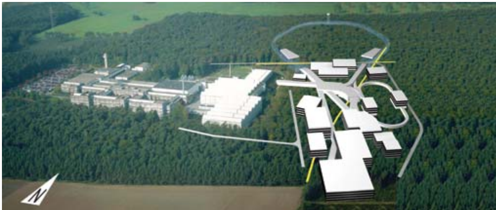
Fig. 15. The accelerator complex for Antiproton and Ions at GSI. Left: the existing facilities; right: artistic view of the new facility (FAIR). In light blue is visible the footprint of the ring that hosts SIS100 and SIS300 accelerators.
