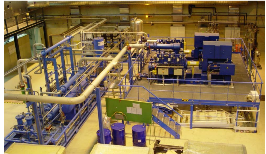
1.5 kW @ 4.5 K helium refrigerator
