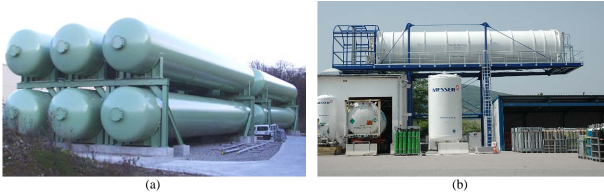
Fig. 5. Helium storage at LHC: 250 m 3 medium-pressure helium storage tanks (a) and 120,000 l liquid-helium reservoir (b).
