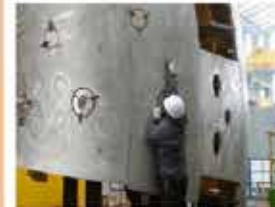
Fit-up for welding of 8 keys
