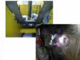
In & outside welding
