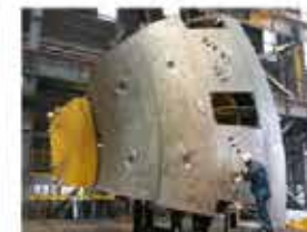
Fit-up for welding of 6 keys
