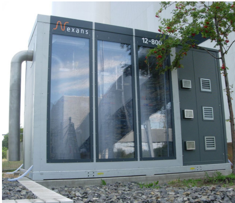
Figure 7. Completed FCL of Project 2 after installation in the power plant.
