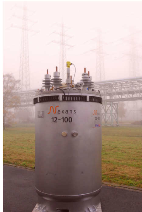
Figure 6. Completed FCL cryostat of Project 1.
