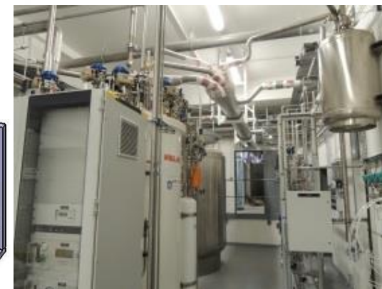
Cryogenic satellite (-271°C) and cryoline (caloduc)
