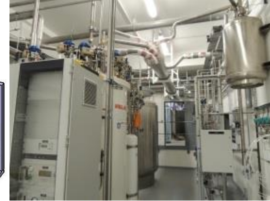
Cryogenic satellite (-271°C) and cryoline (caloduc)
