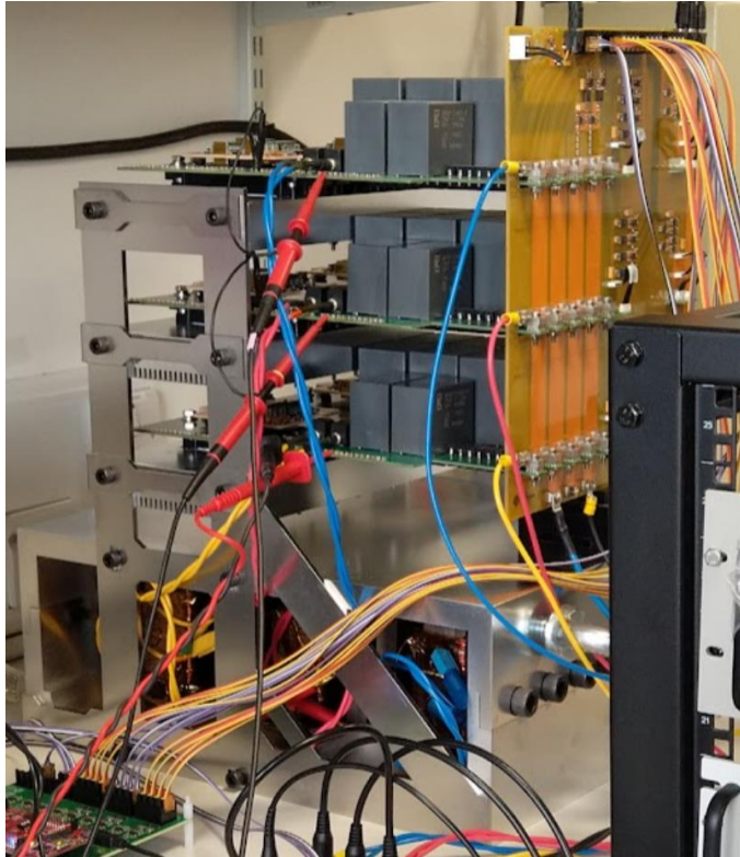
100 kW cryogenic inverter
