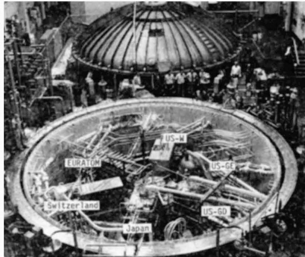
Photo. 2 Six LCT coils installed in vacuum tank: October 1985
