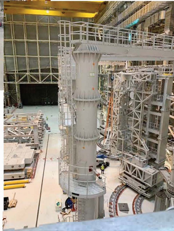
Main assembly hall June 2020 Sub Sector Assembly Tools (SSAT) Each for mounting 2 TF coils and 1 VV sector
