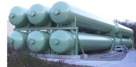
Gaseous helium storage 250m 3
