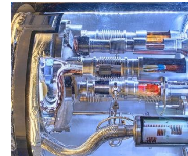
LHC magnet interconnection
