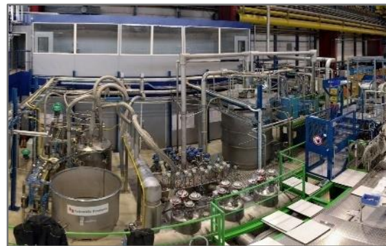
Cryogenic infrastructure in B180
