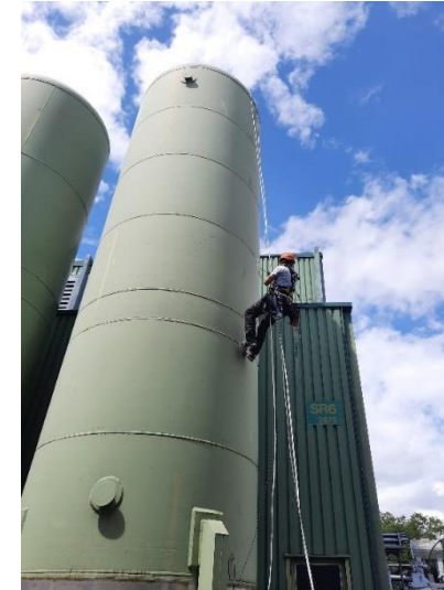
Acoustic emission requalification of pressure vessels
