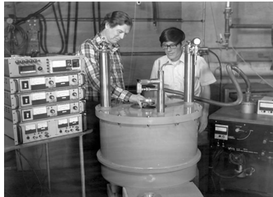
Fig. 15. System for 95 GHz Gyrotron.
