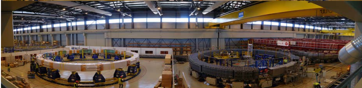
PF coil impregnation
