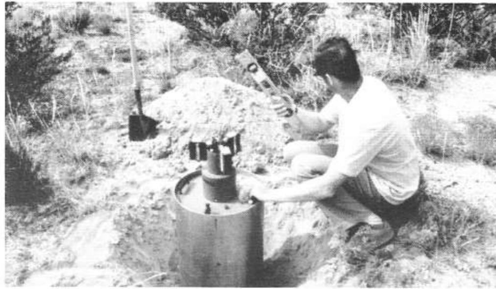
Installation of SQUID magnetometer, which involves leveling and partial burial to prevent wind vibration
