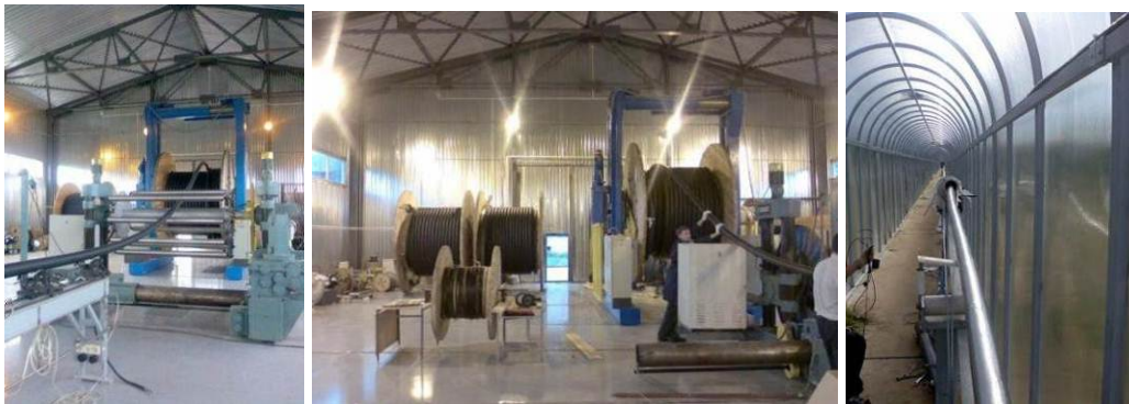
Fig. 3. Insertion HTS cable into cryostat by pulling through method.
