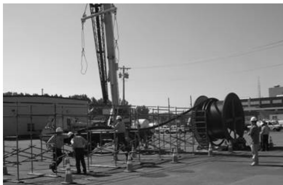
Fig.15. Installation of the 30 m long cable made by Sumitomo Electric with nearly 10,000 m of SuperPower's 2G HTS wire.
