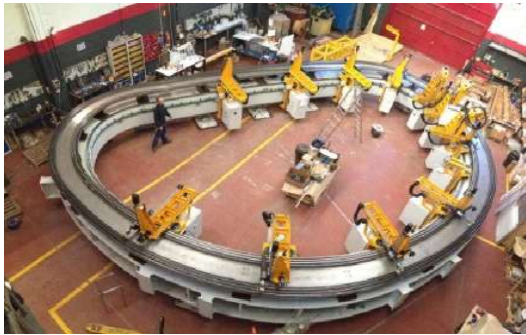
DP Turn Insulation inside Radial Plate
