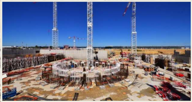
Plexiglass Formwork for Bioshield Construction (3.2 m thick walls)
