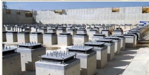
Tokamak Building Pit and Foundation (17 m deep; 120 x 90 m)
